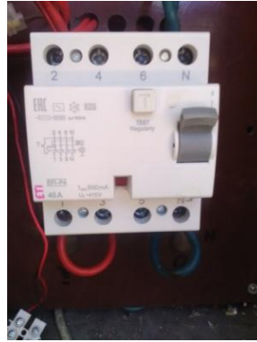
Figure 9 – Actual Appearance of an RCD (FID Switch)
